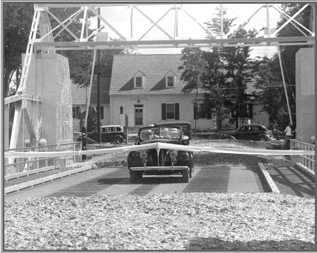
Lafayette Street Bridge - May 1937
