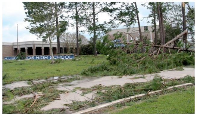
Building Damage Downed trees from Hurricane Gustav at H.L. Bourgeois High School. Photo Credit: FEMA/Jacinta Quesada
