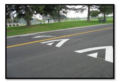
Speed humps are raised curved traffic calming devices that are 12 feet long, and 3 to four inches high. They reduce traffic by 40-60% and reduce the number of collisions on a street. Speed humps are the preferred alternative to speed bumps since they are less likely to damage vehicles or contribute to road departures due to their size and shape.
