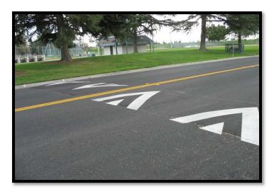
Speed humps are raised curved traffic calming devices that are 12 feet long, and 3 to four inches high. They reduce traffic by 40-60% and reduce the number of collisions on a street. Speed humps are the preferred alternative to speed bumps since they are less likely to damage vehicles or contribute to road departures due to their size and shape.
