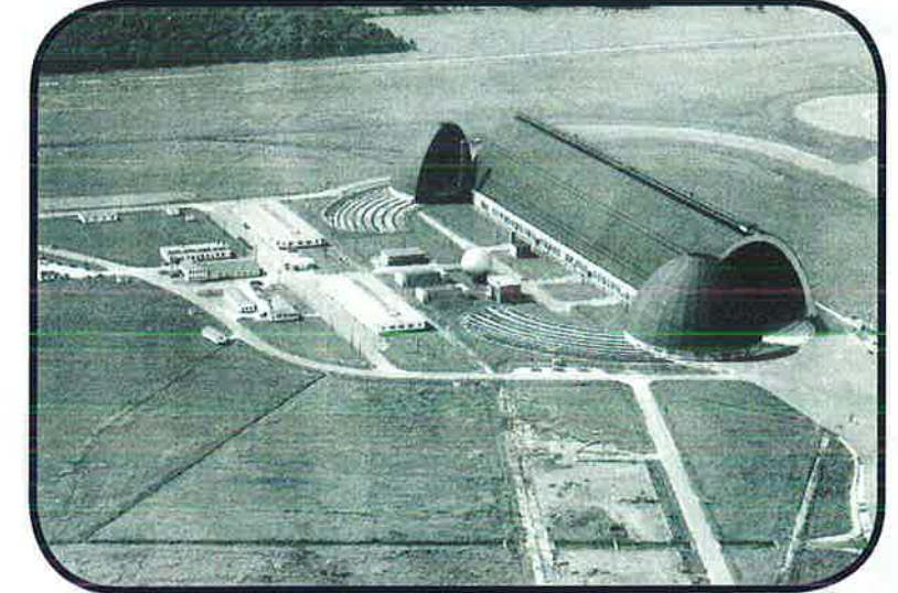
HISTORIC PHOTO OF BLIMP HANGAR AT HOUMA BASE
